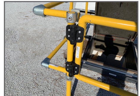
Rugged hinges allow gate tension adjustment.
